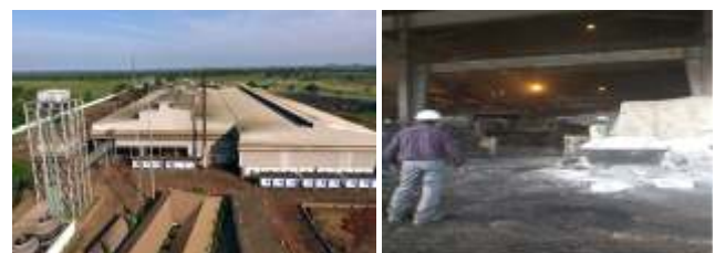
Aerial of the Plant
